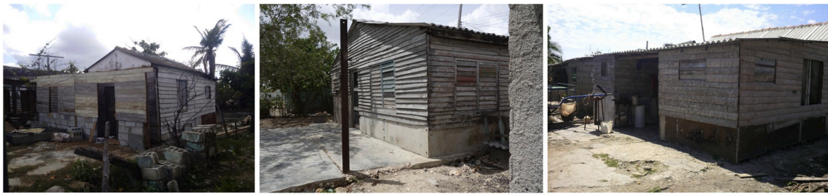
Fig. 6. Reinforced columns and sidewalls of houses in Carahatas.
